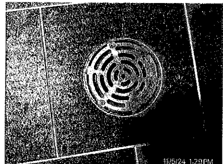
FD to be cleaned on inside
