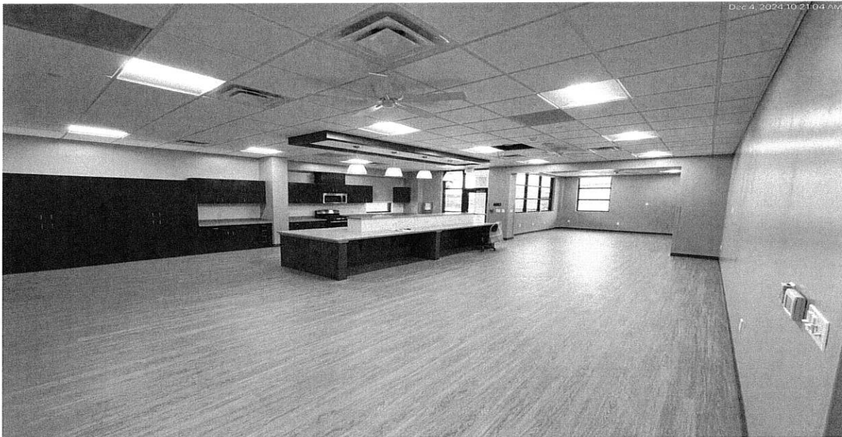
12/4/24 Finished kitchen area
