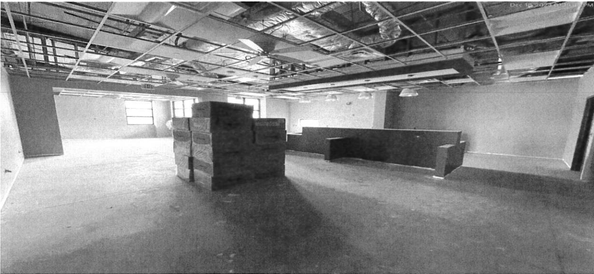
12/18/24 Building interior progress
