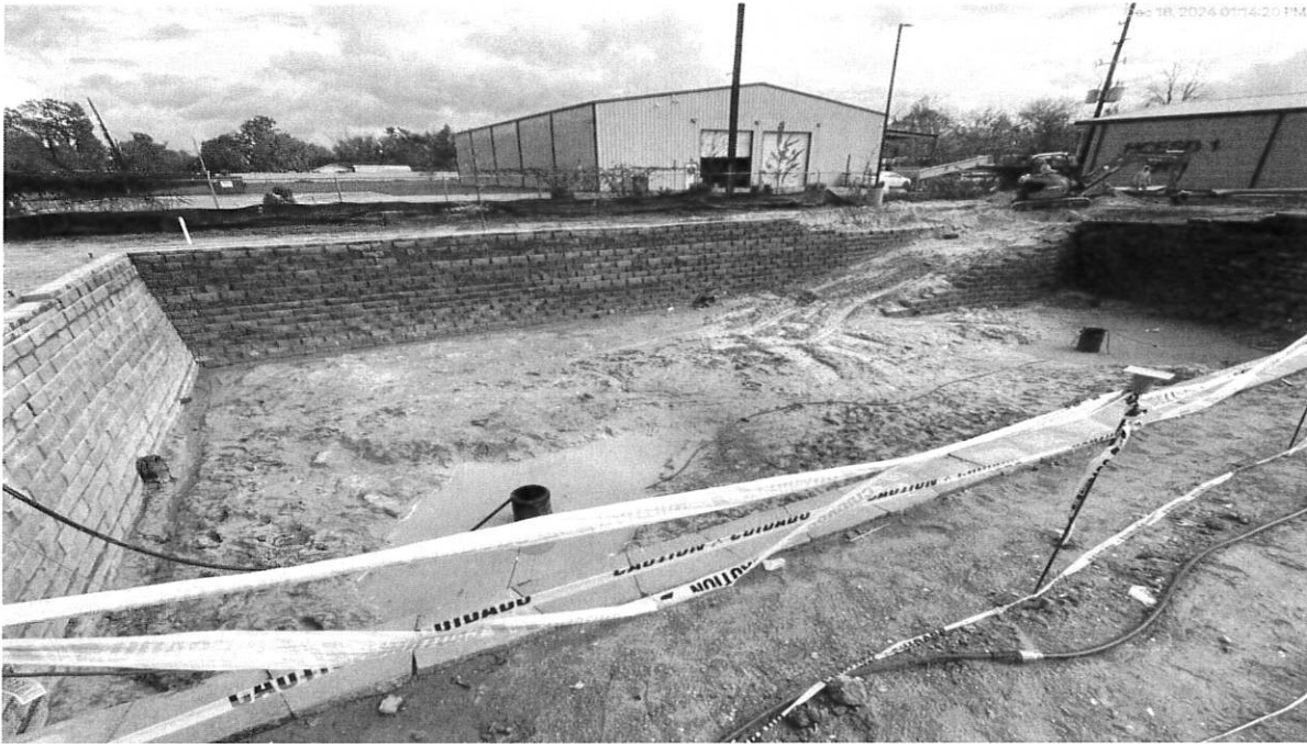
12/18/24 Pond re-work prepping commencement
