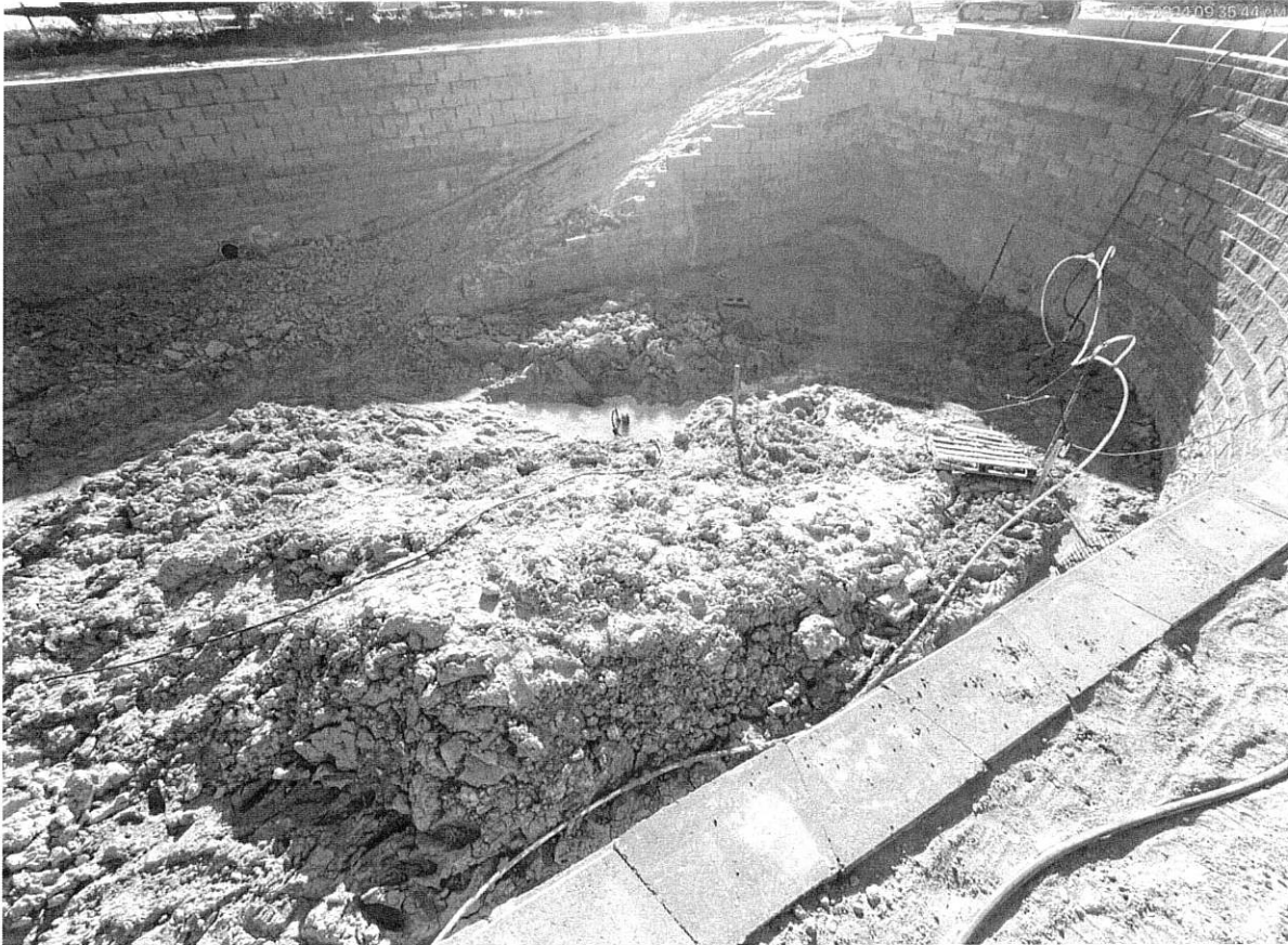
10/18/24 Pond drying status
