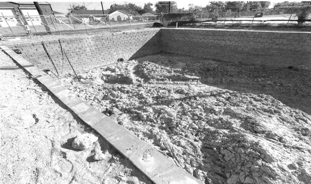
10/18/24 Pond drying status
