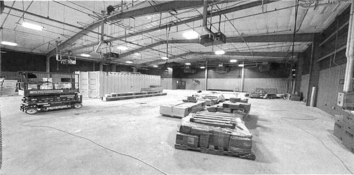
10/9/24 Apparatus bay progress
