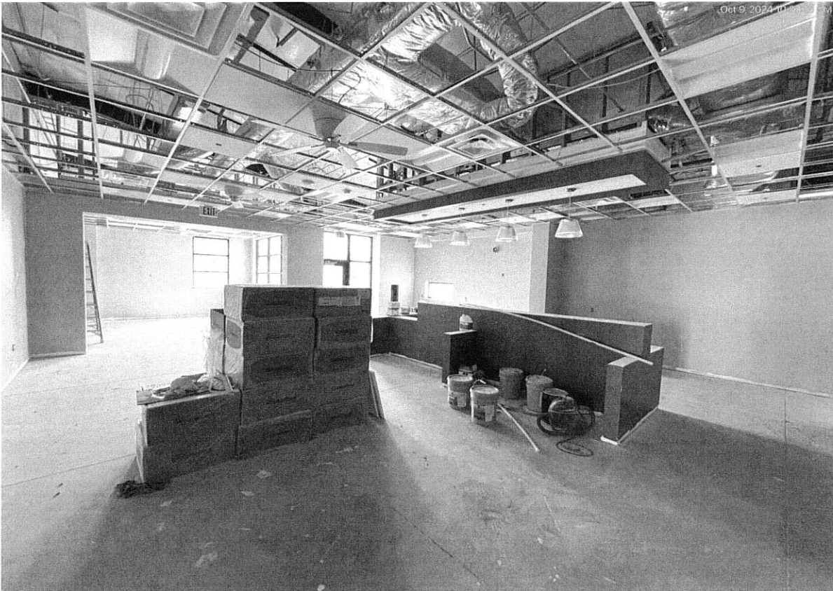
10/9/24 Kitchen area progress
