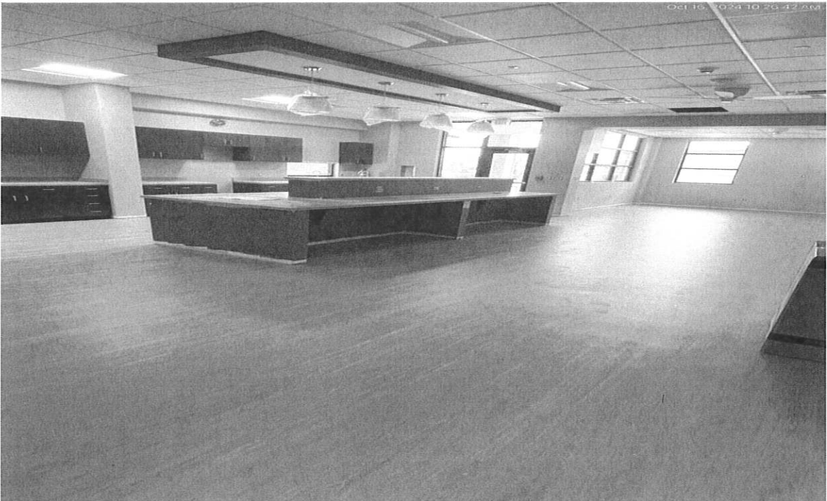
10/16/24 Kitchen area progress
