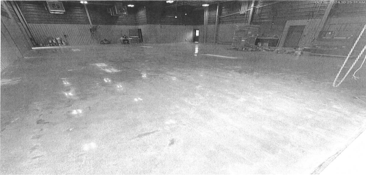
10/16/24 Apparatus bay polished concrete underway
