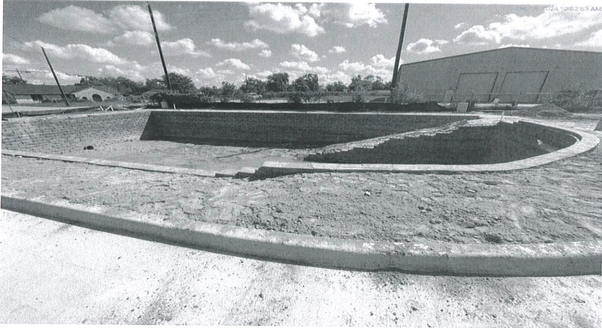
9/19/24 Detention pond after pumping water out
