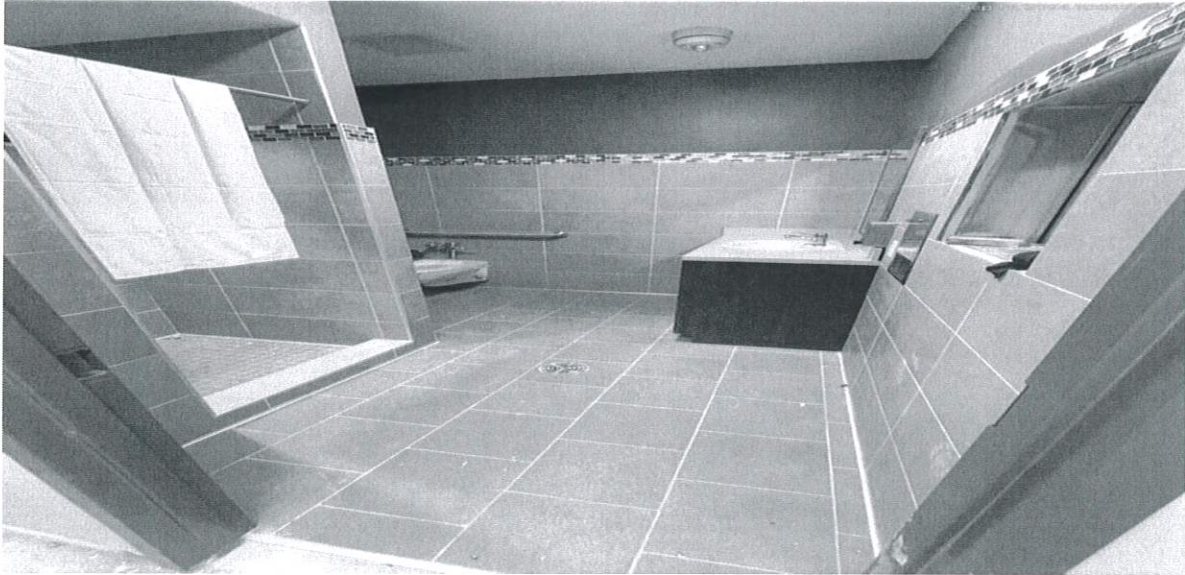
9/19/24 Typical restroom progress
