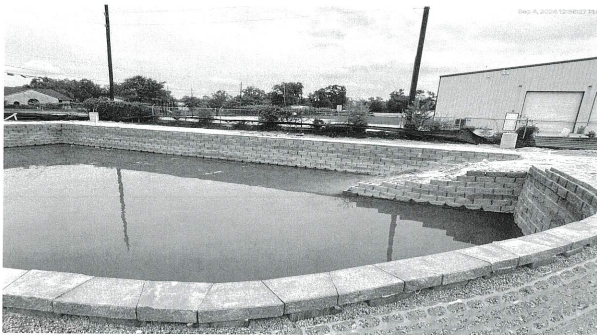
9/4/24 Detention pond beginning of the month
