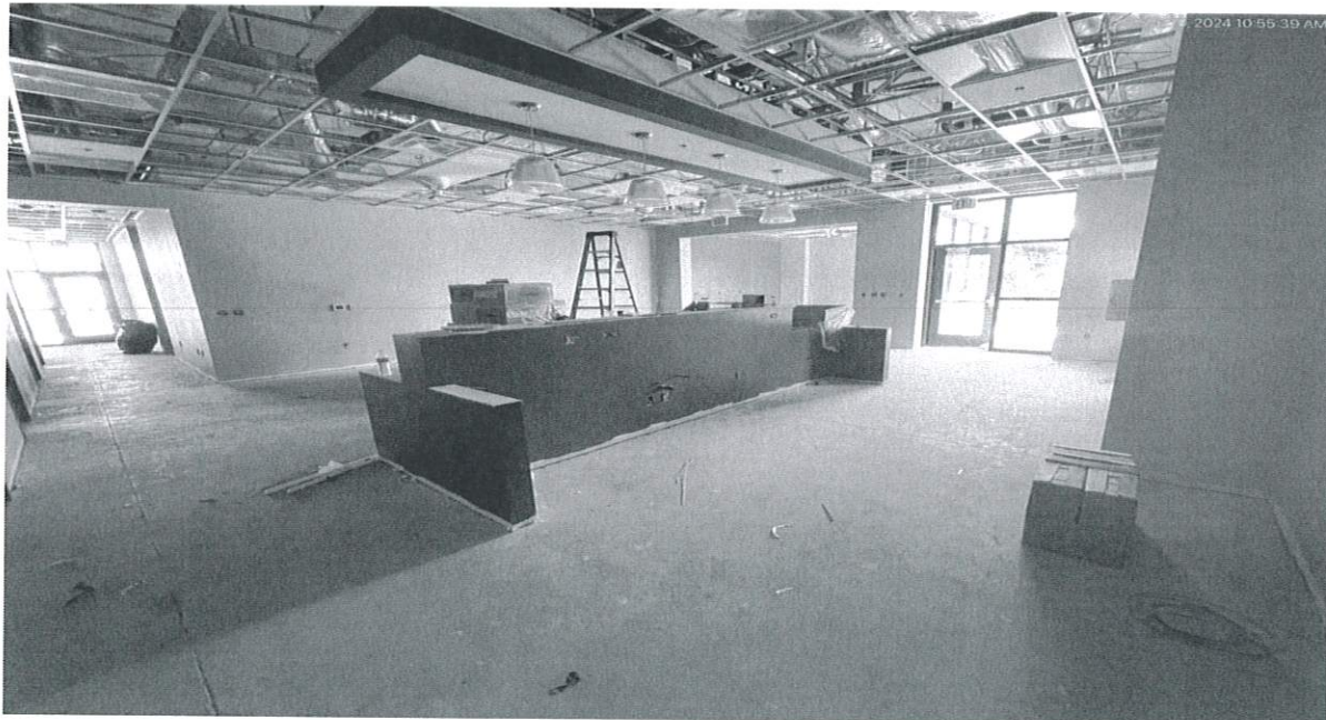
9/19/24 Kitchen area progress
