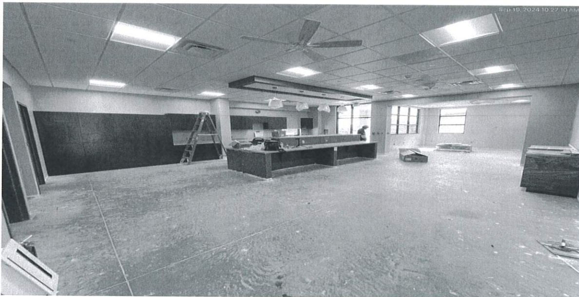
9/19/24 Kitchen area progress
