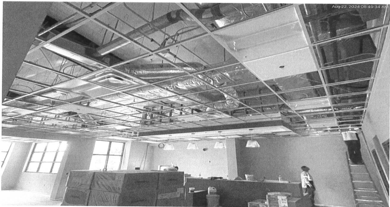
8/22/24 Kitchen area progress
