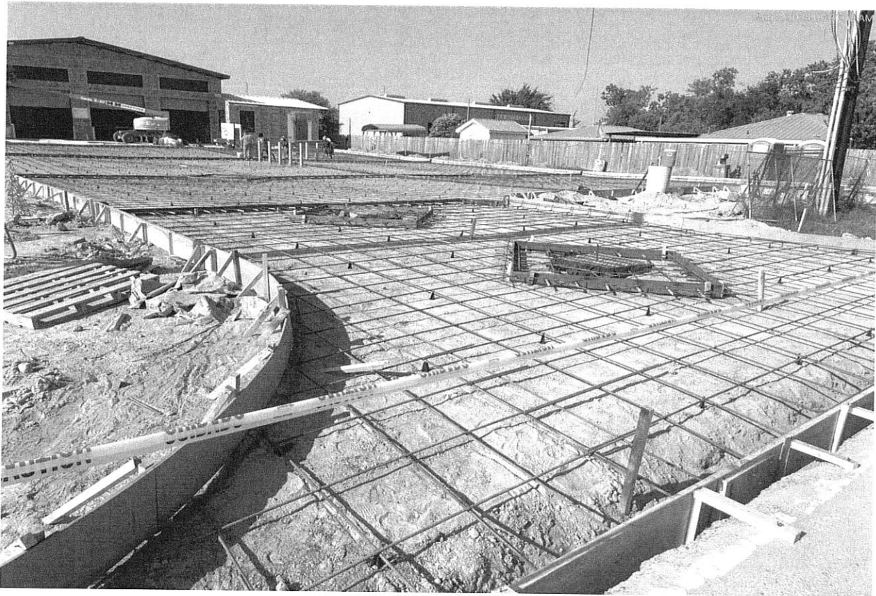
8/8/24 Paving forms/rebar installation underway
