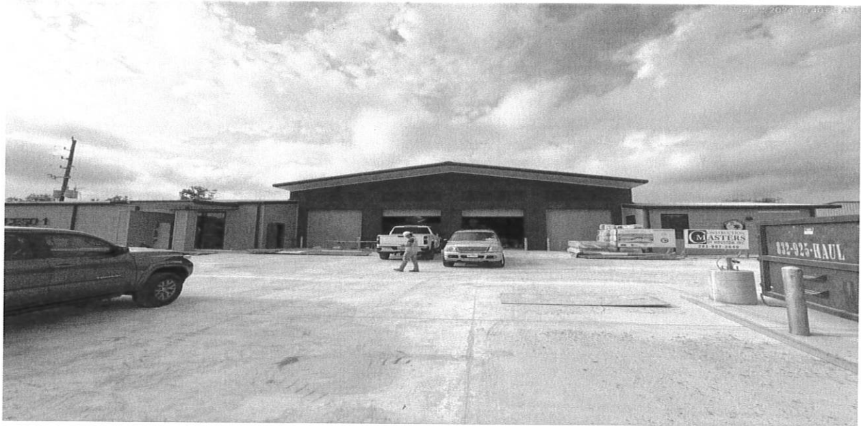
8/22/24 Building exterior progress
