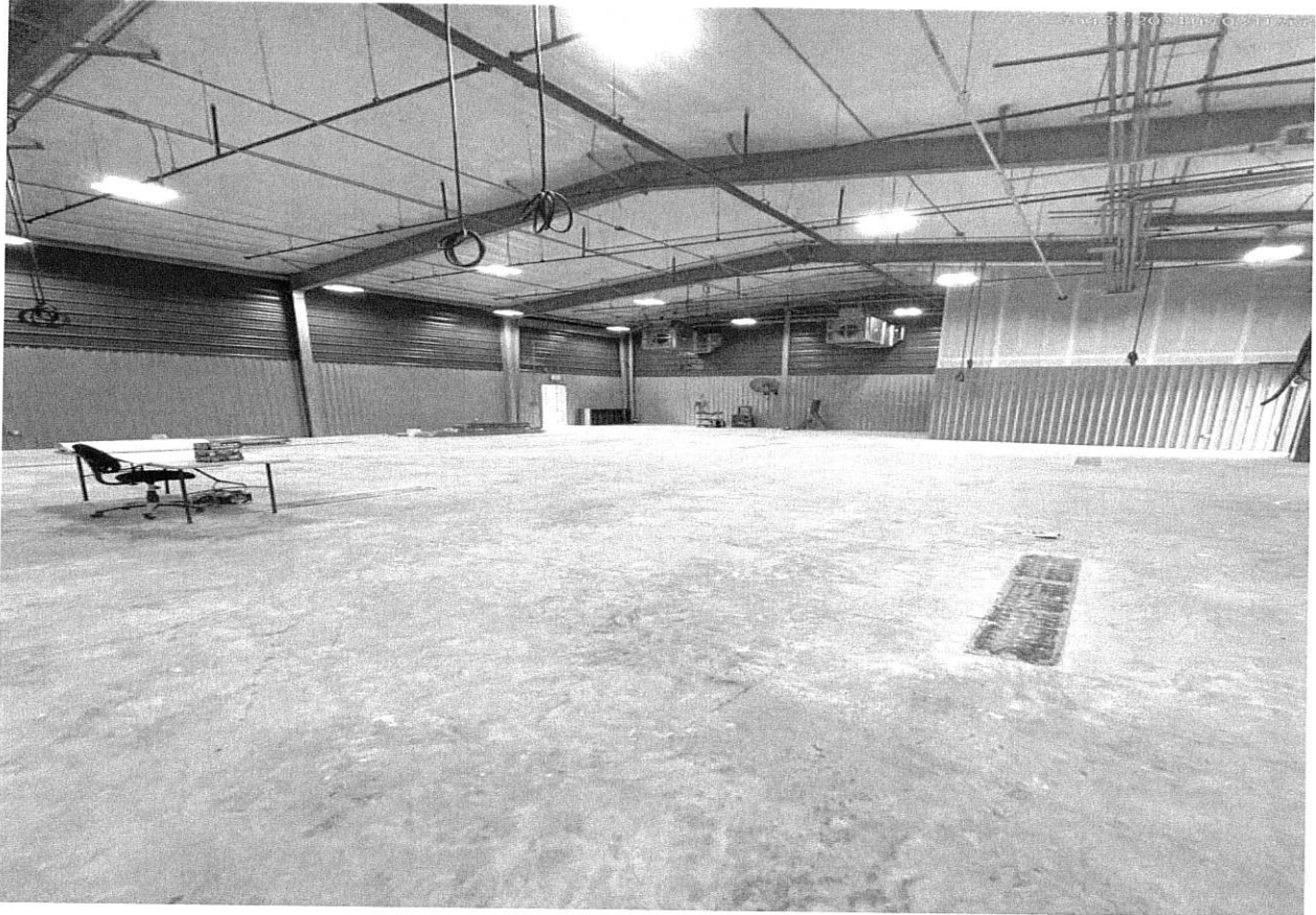
8/22/24 Apparatus bay progress
