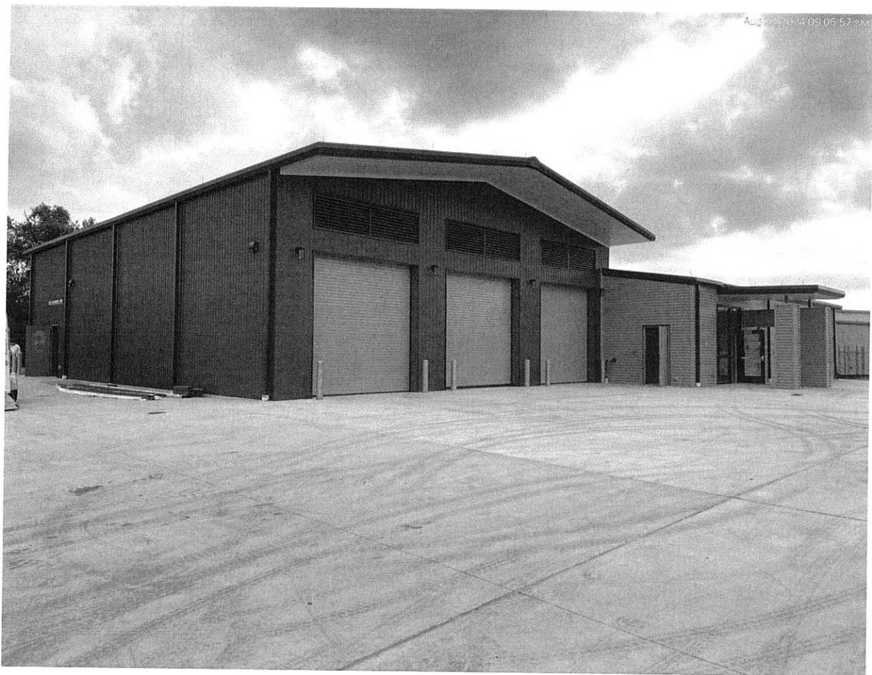
8/22/24 Building exterior progress
