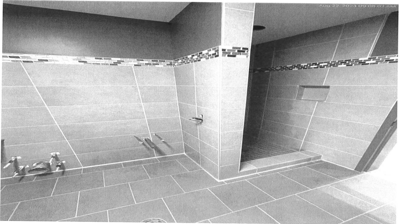
8/22/24 Typical bathroom progress
