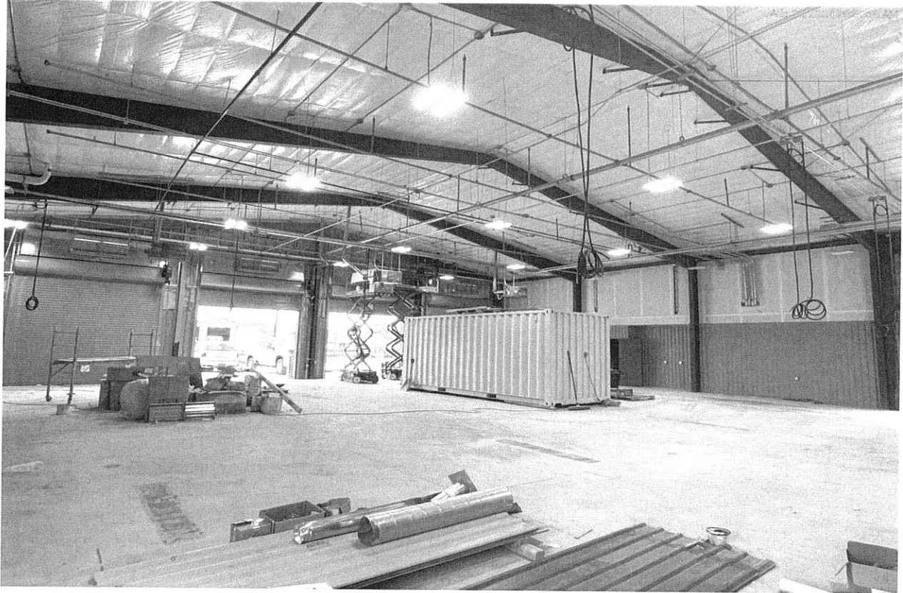
8/22/24 Apparatus bay progress
