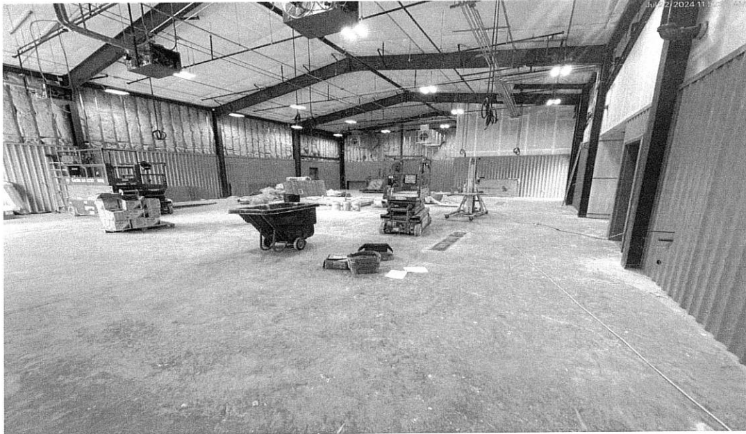
7/22/24 Apparatus bay progress
