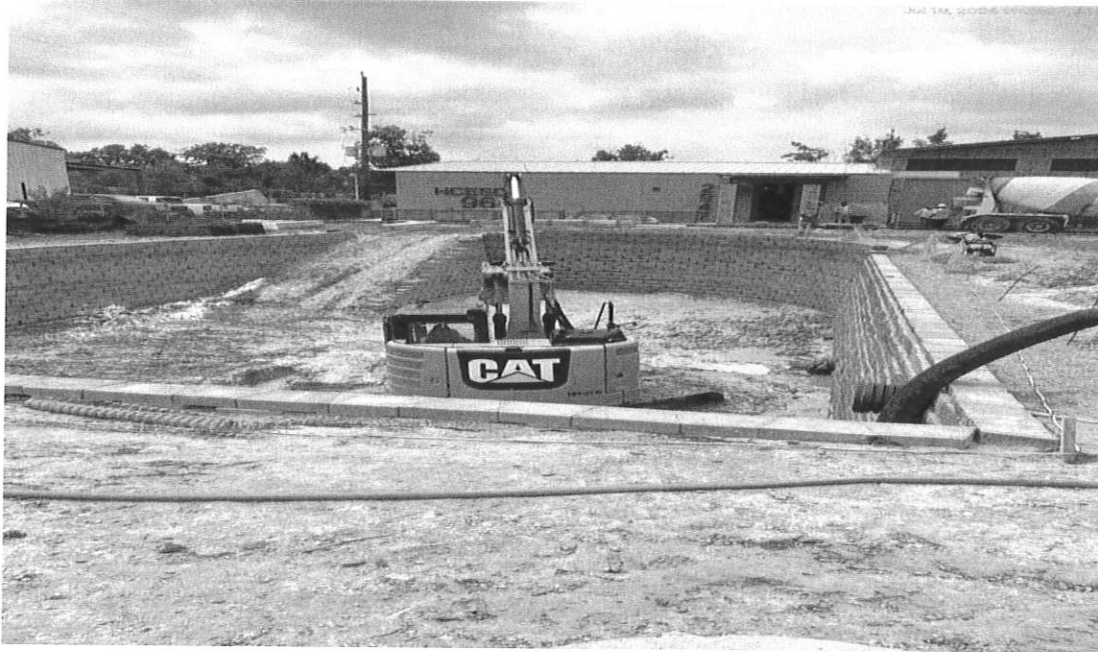
7/19/24 Detention pond progress
