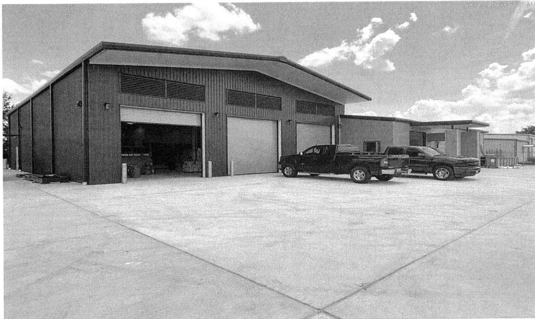
7/22/24 Front building progress
