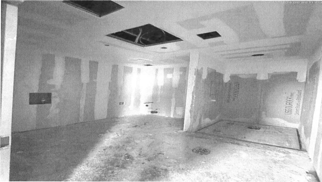
7/23/24 Dorm restroom progress
