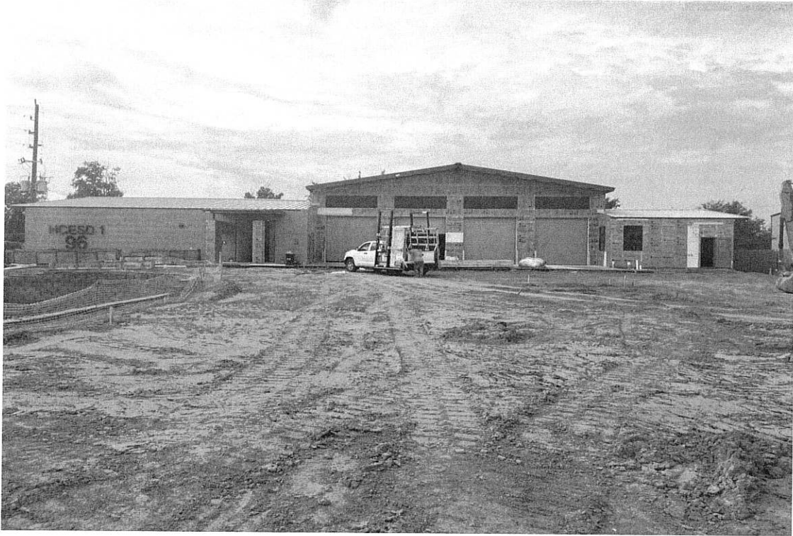
7/23/24 Building exterior progress
