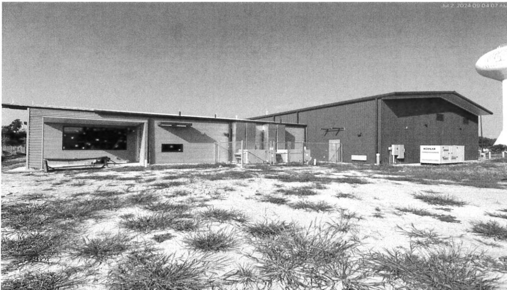
7/2/24 Rear building progress
