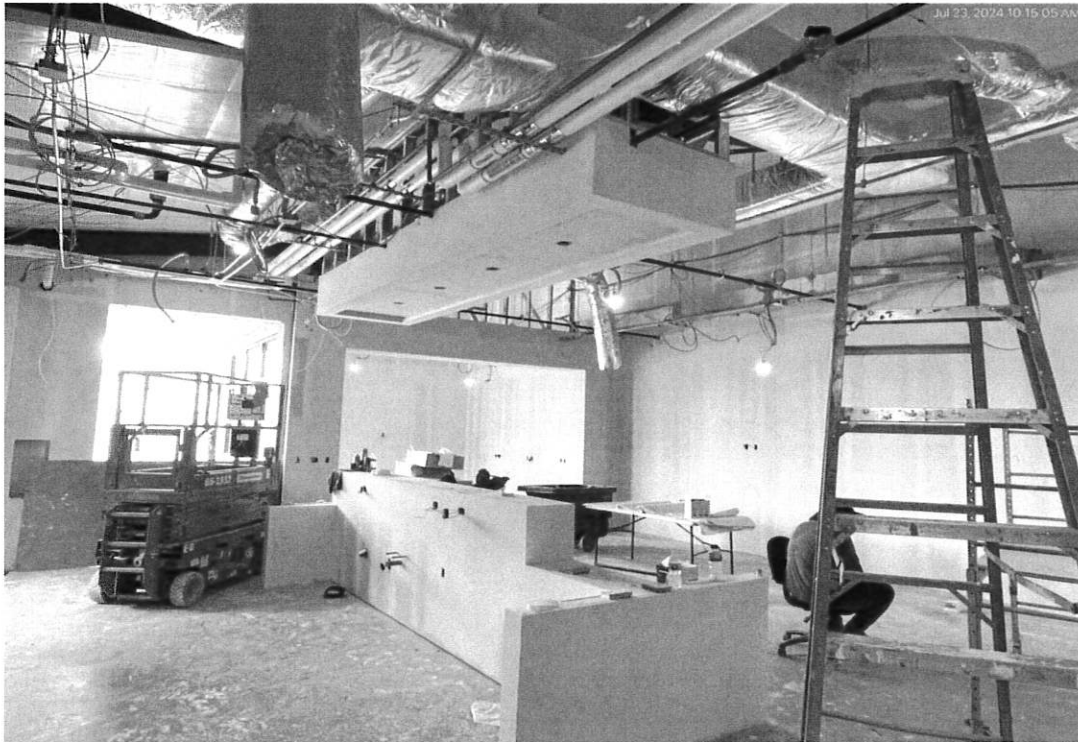
7/23/24 End of month kitchen progress
