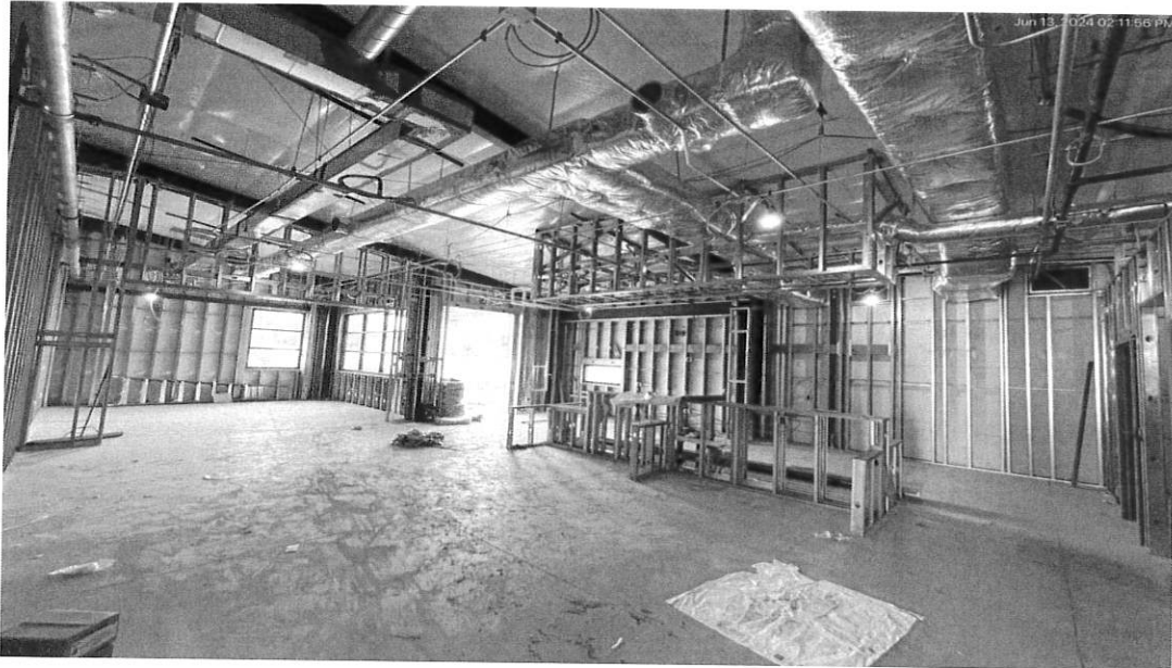
6/13/24 Kitchen area progress
