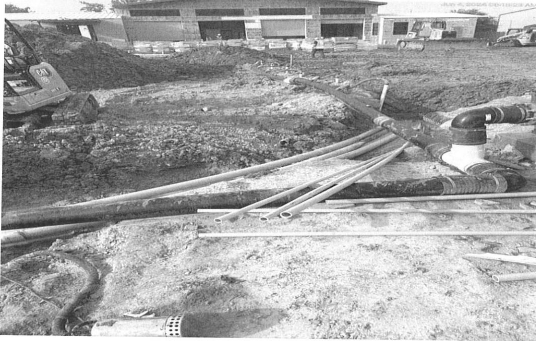
6/4/24 De-watering and pond excavation underway
