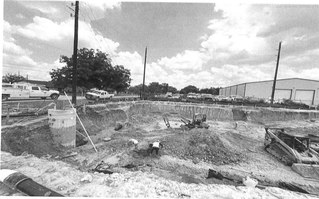
6/13/24 Pond excavation and utilities installation underway
