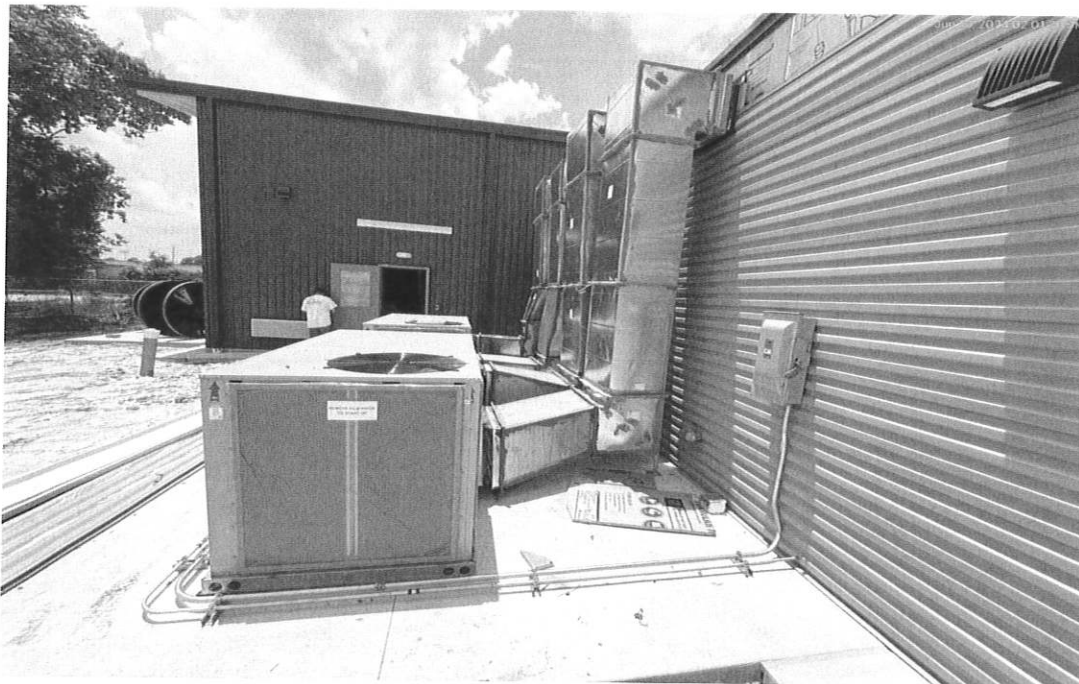
6/13/24 AC units' installation complete
