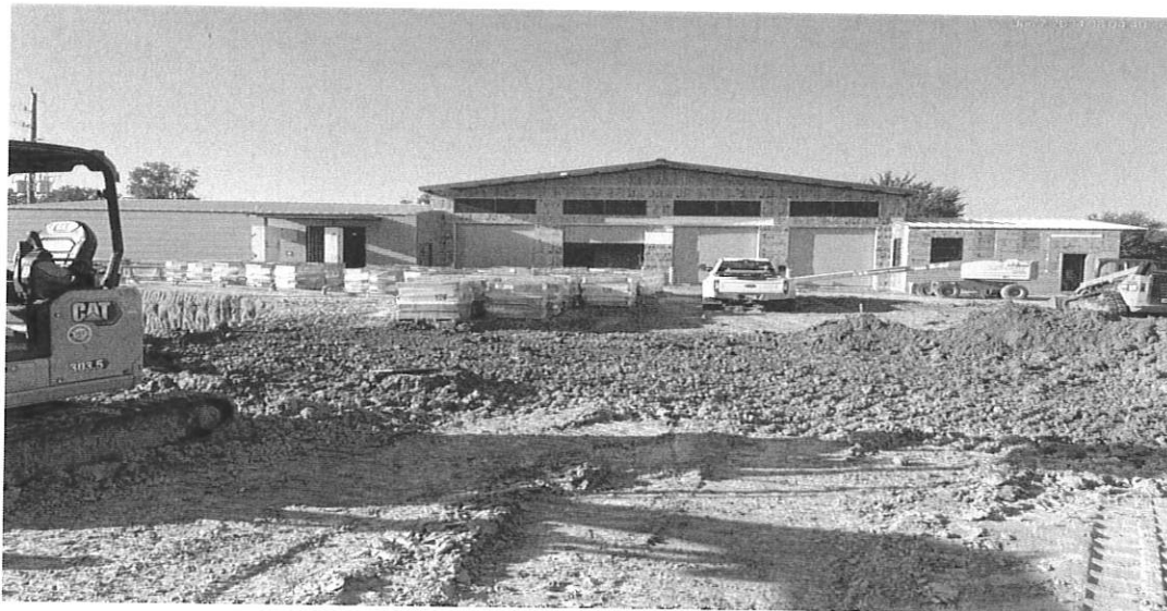
6/7/24 Building exterior overview
