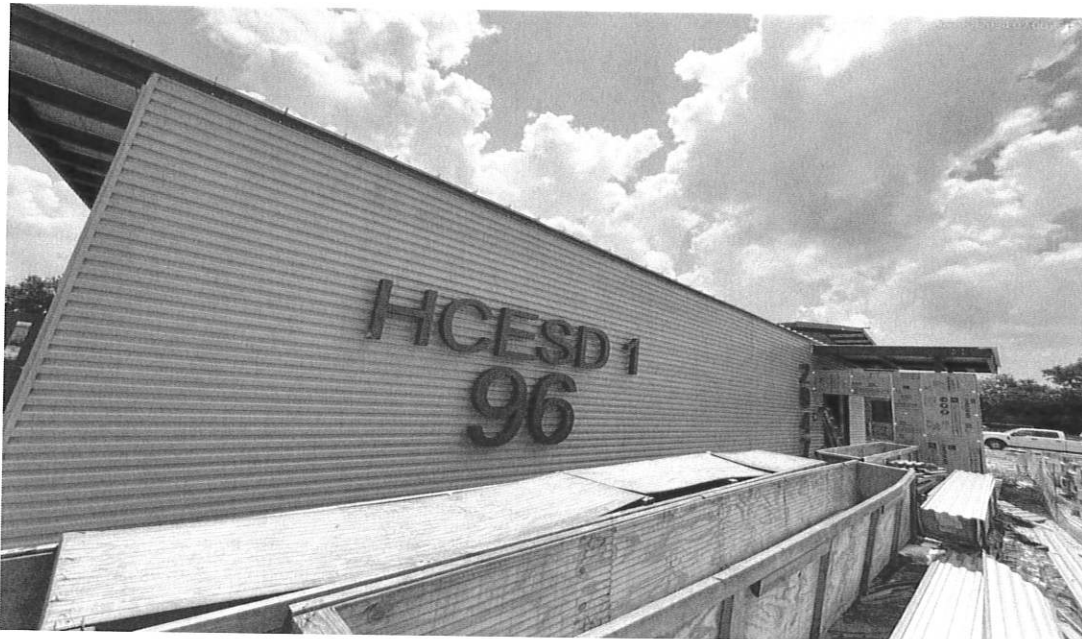
6/13/24 Exterior signage installation underway
