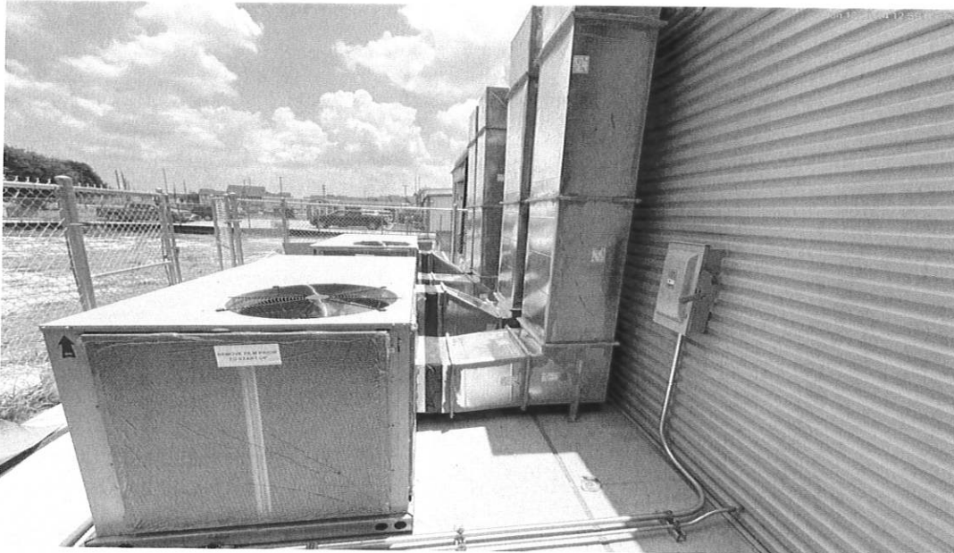
6/13/24 AC units' installation complete
