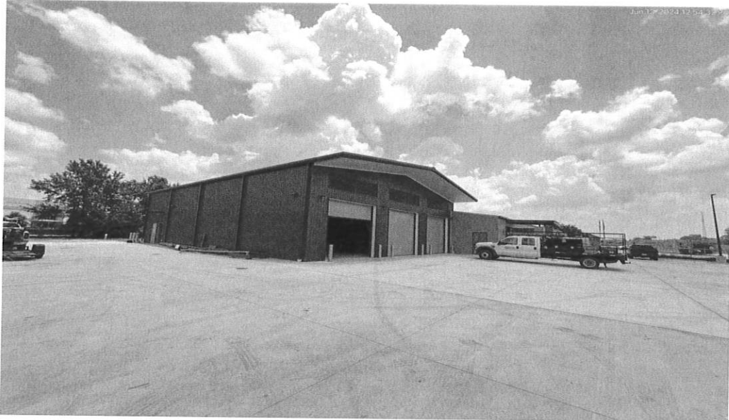
6/13/24 Building exterior overview
