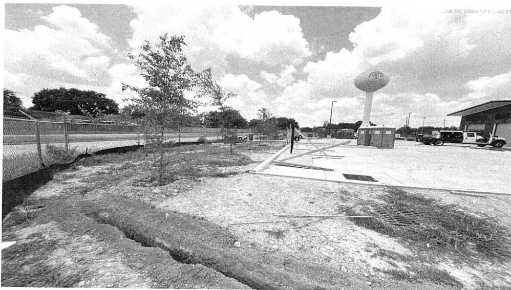
6/13/24 Landscaping and irrigation underway
