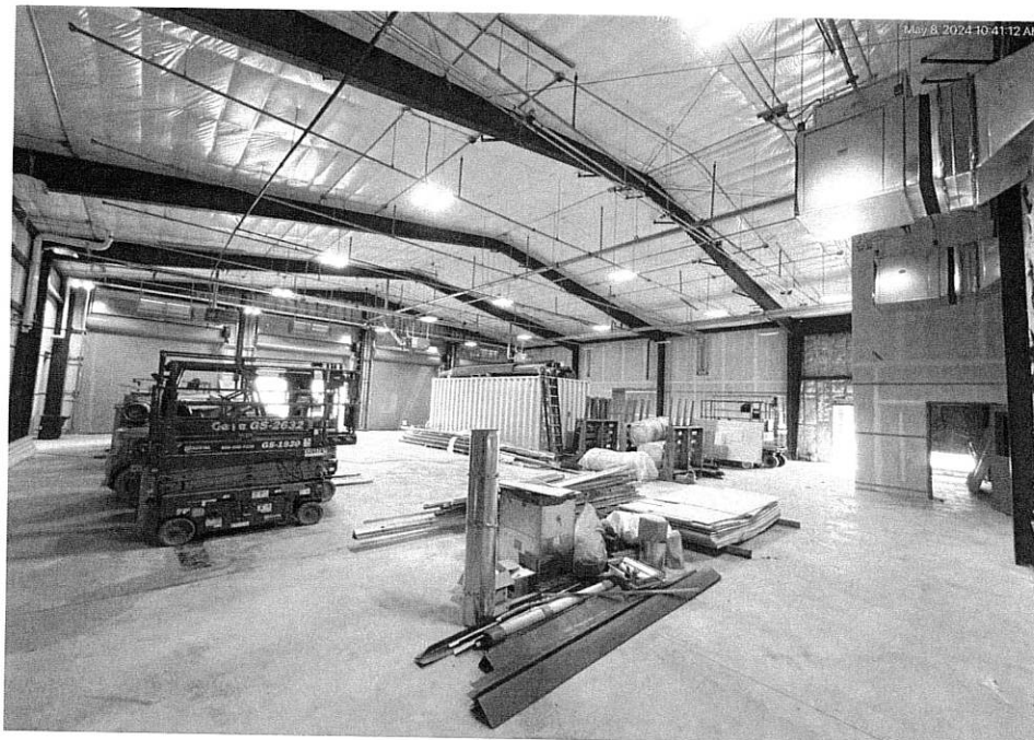
5/8/24 Apparatus bay progress
