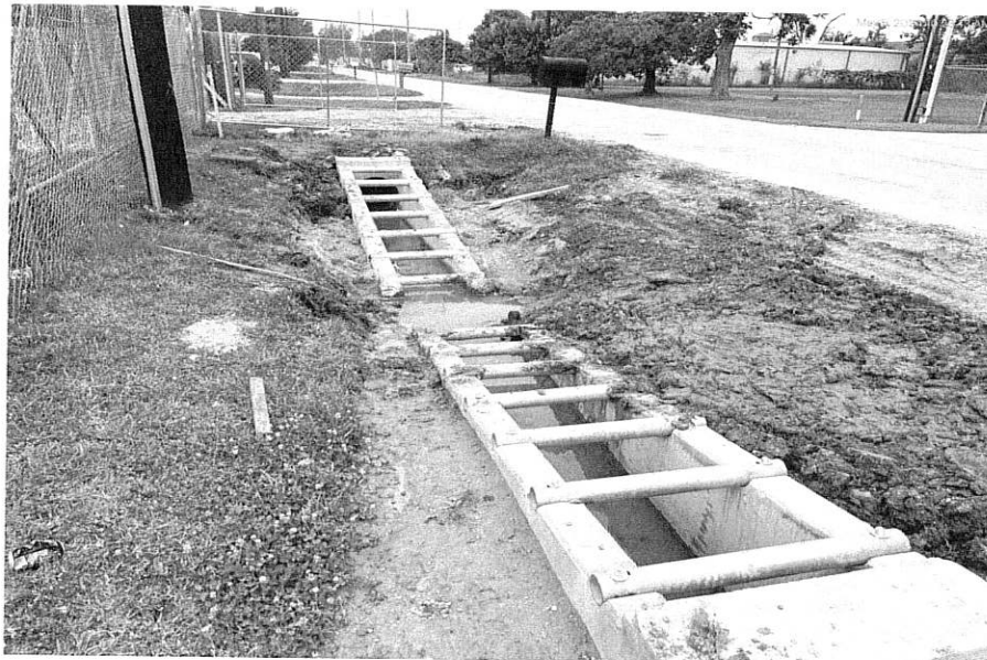
5/8/24 Entry culverts installed
