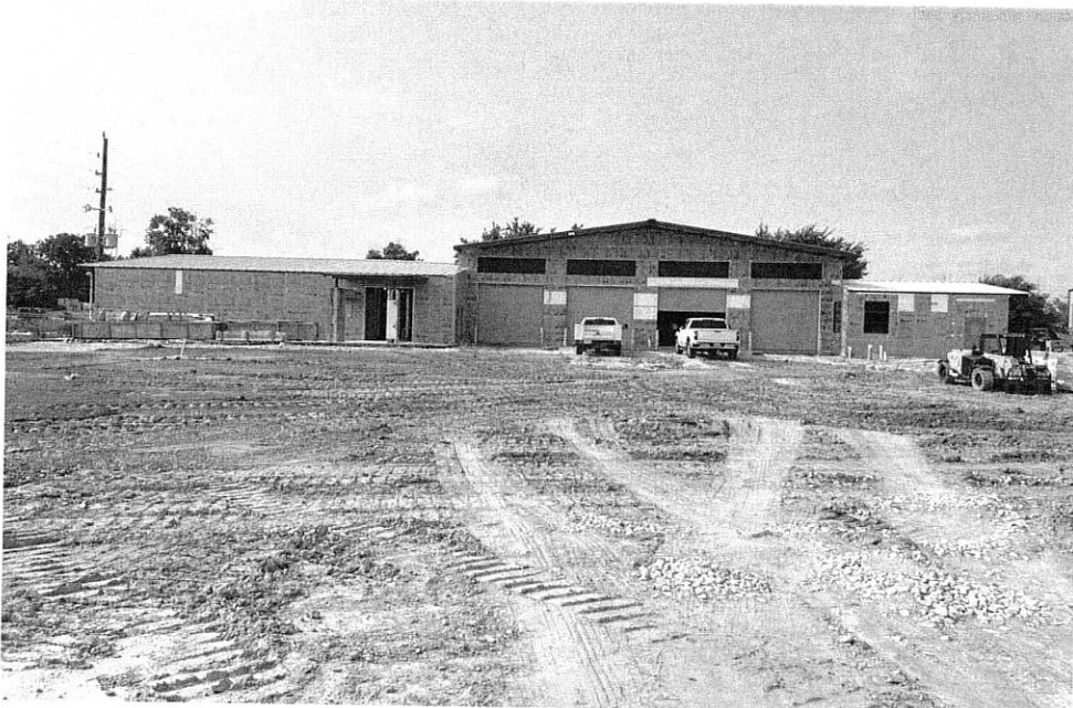
5/16/24 Site and building overview
