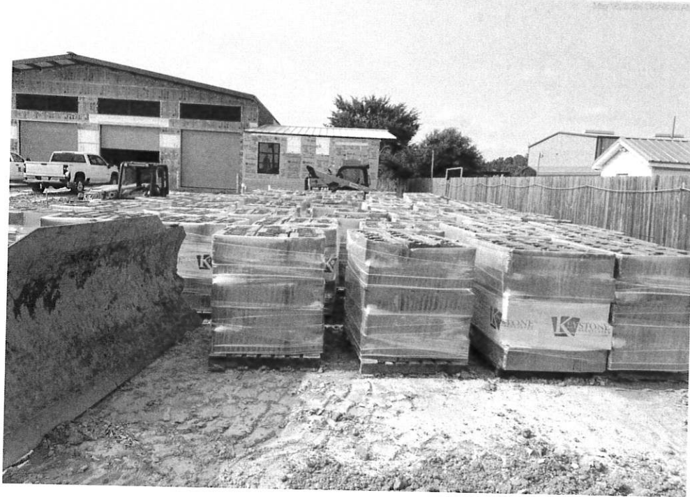
5/16/24 Detention pond retaining wall materials onsite
