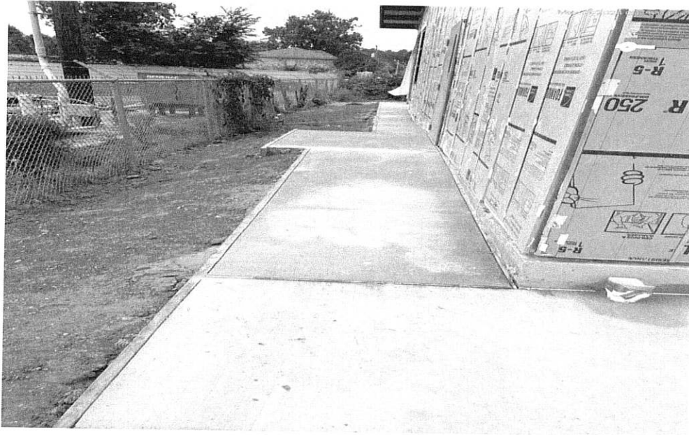
5/13/24 Sidewalks and mow strips poured
