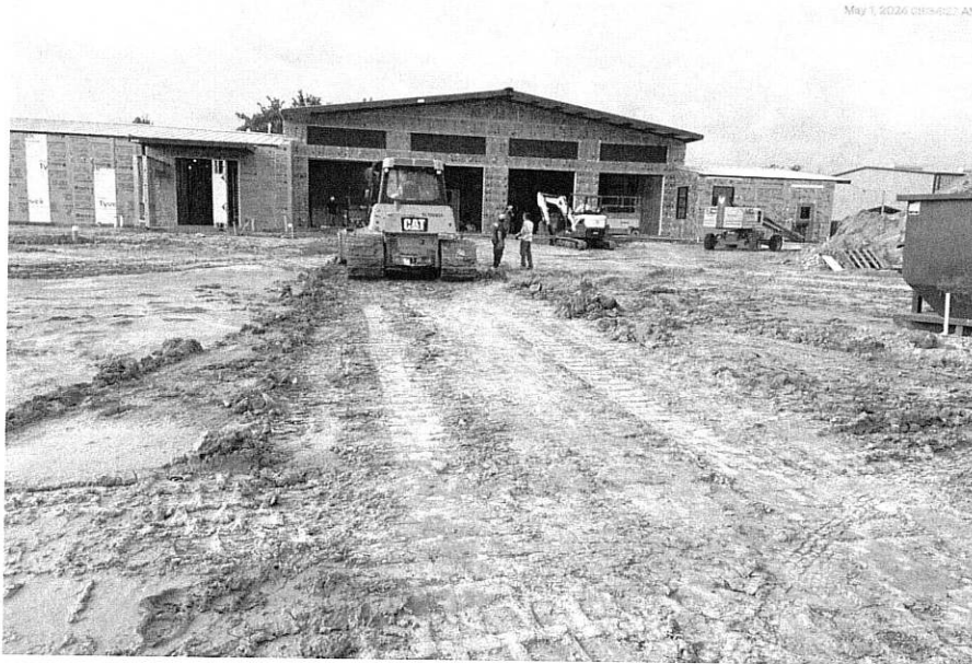
5/1/24 Site grading and site utilities installation underway
