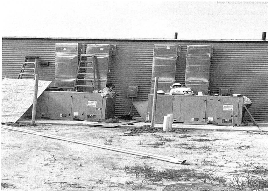
5/16/24 Mechanical equipment installation underway
